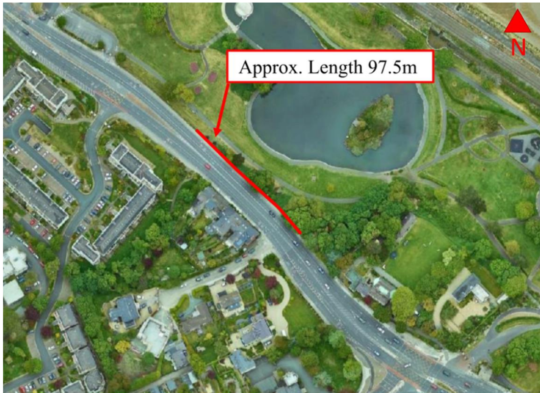
Figure 8.1: Location of principal retaining wall
